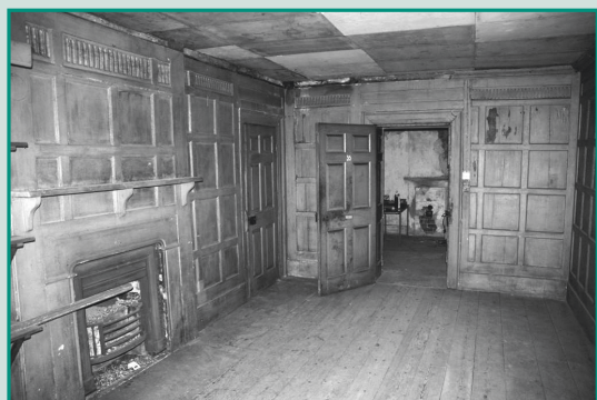
One of the panelled rooms in the attic area.
